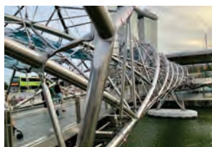
Helix Bridge, Singapore(2009)
