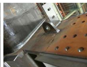
06_Welding against earthquake
